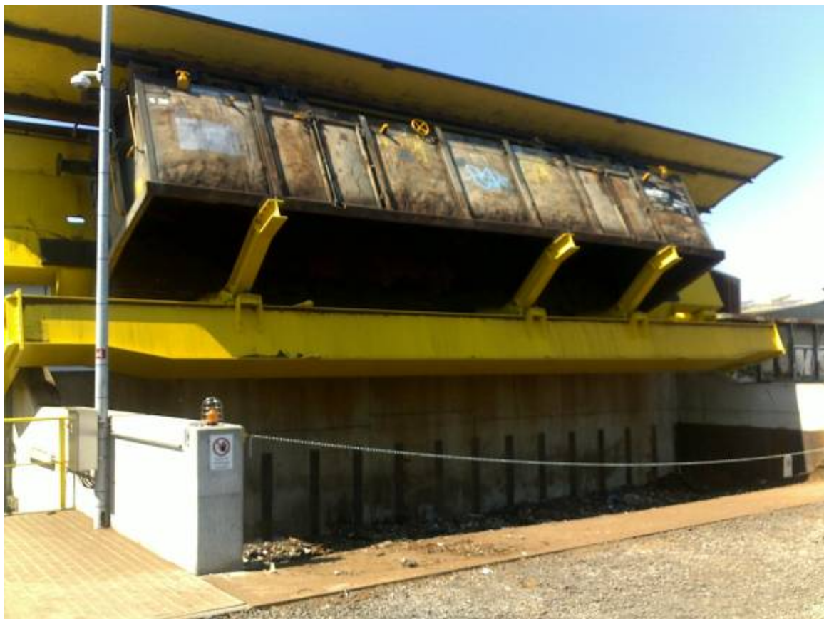
Picture 4: Wagon fully tilted, vibrator active, dirt falling in bunker
