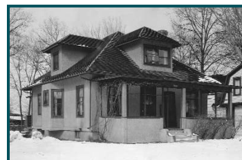
◀ 3817 Thomas Ave., built 1904
