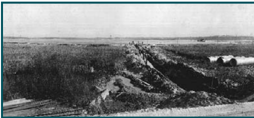
▲ Storm sewer excavation at Lake Calhoun
