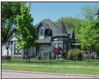
Historic home in north residential district
