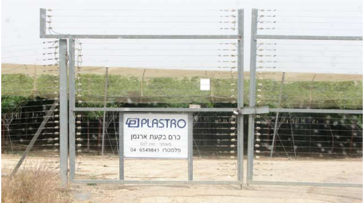
This fence is part of an electronic fence system placed by the Israeli authorities around an area of about 770 dunam cultivated by the settlers of the Argaman settlement in the Jordan Valley.
