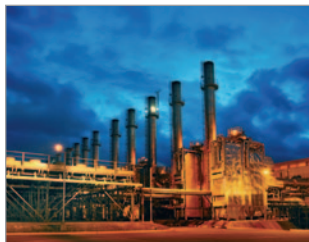
Turnkey Power Plants (MAN Diesel & Turbo)
