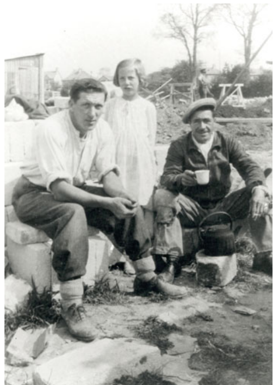
Downham Estate Under Construction, Downham, Lewisham, c.1925
