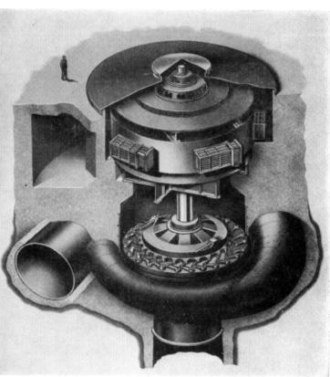
This is an artist's drawing of the largest electric motor and reversible pump-turbine ever built. The equipment, which is being built by Allis-Chalmers, will be the heart of a pumpstorage project at Hiwassee Dam in southwestern North Carolina on the TVA's power network. It is scheduled for completion in 1955.
