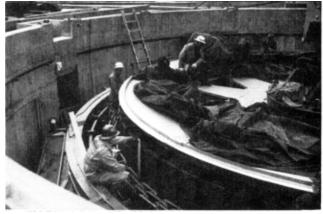
CRUSHING STICKS of ¼-inch plywood, held in the ½-inch air gap between the stator and rotor pole faces, assured proper centering of the rotor as it was lowered. (FIGURE 8)
