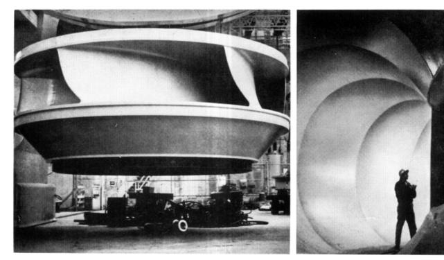
WHEN WEAR RINGS were fitted onto this 266-inch diameter three-piece runner, strip heaters were used to expand the rings, water spray to contract the runner for the shrink-fit. (FIGURE 4)
