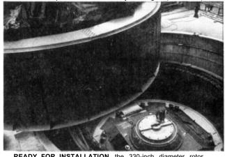
READY FOR INSTALLATION, the 330-inch diameter rotor will be lowered into the 331-inch diameter stator, the expanded keyway mated to the key. (FIGURE 7)
