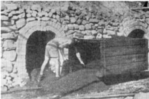
Loading a coke oven at Tivoli
