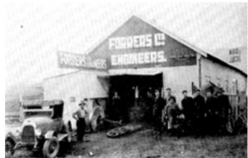
Forrers Ltd, Engineers
