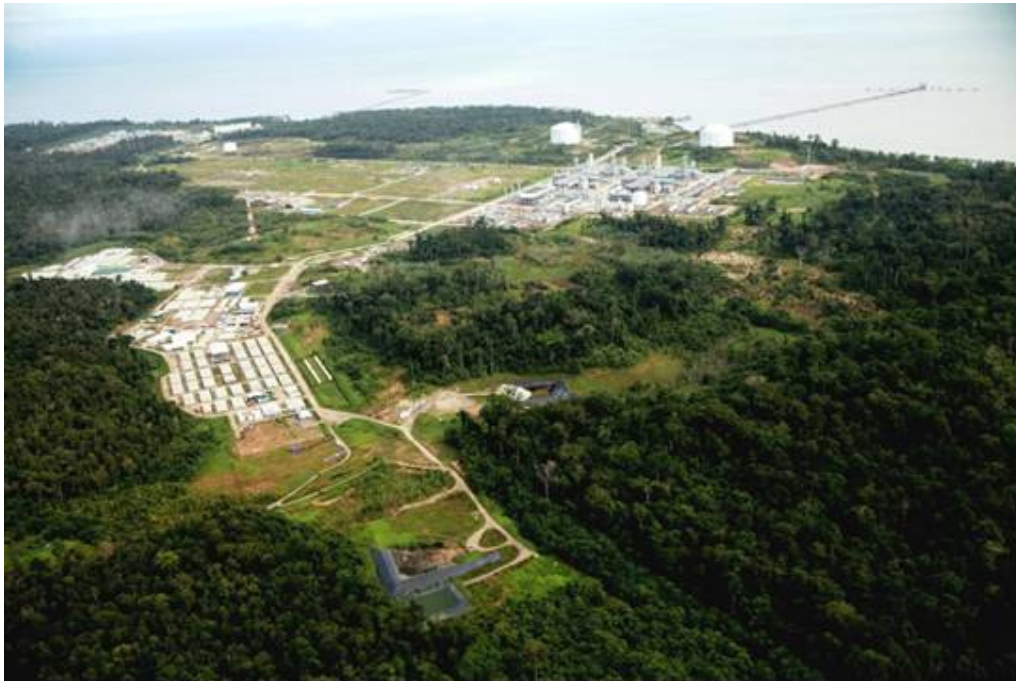
Figure 3: LNG plant and its supporting facilities
