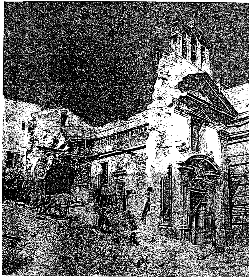
PALERMO, SICILY. SEVERELY DAMAGED BAROQUE CHAPEL.
