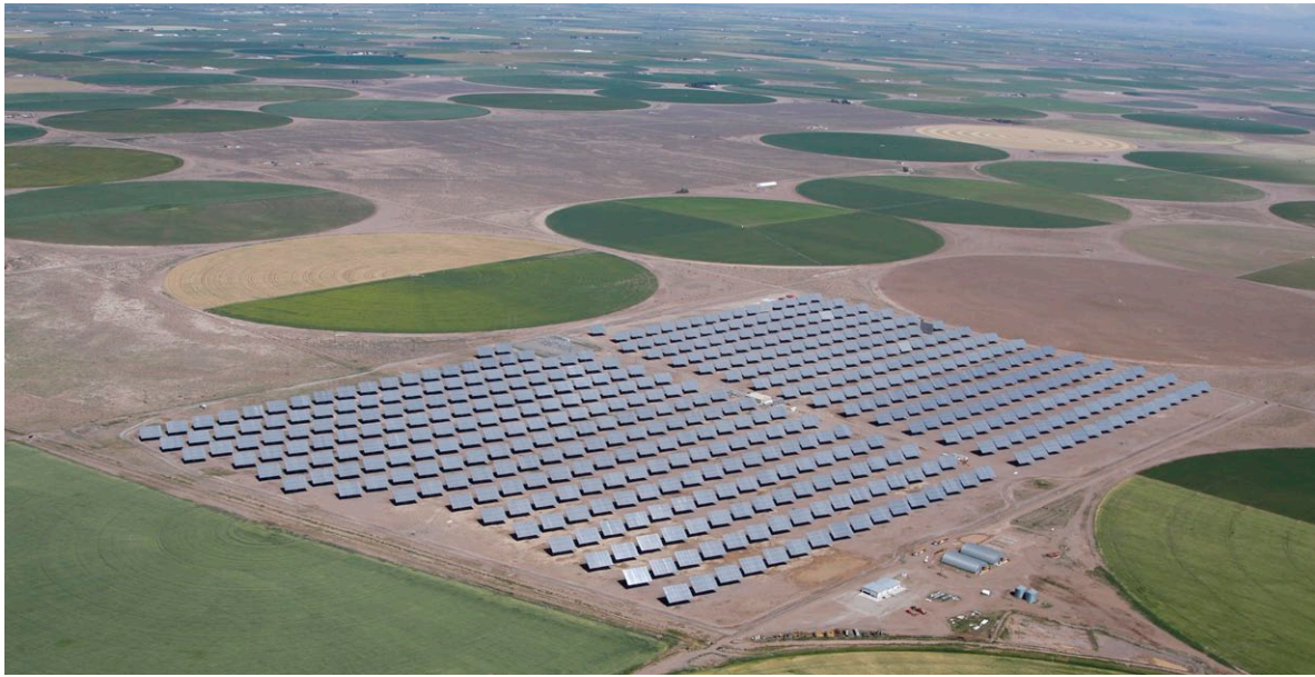
Concentrating PV at Alamosa Solar Farm in Colorado
