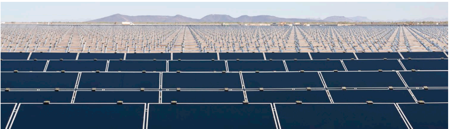
Construction of Agua Caliente Solar Project in Yuma County, Arizona
