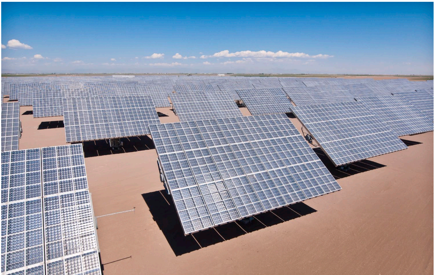
Concentrating PV at Alamosa Solar Farm in Colorado
