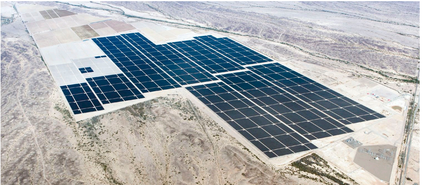
Partially completed Agua Caliente Solar Project in Yuma County, Arizona
