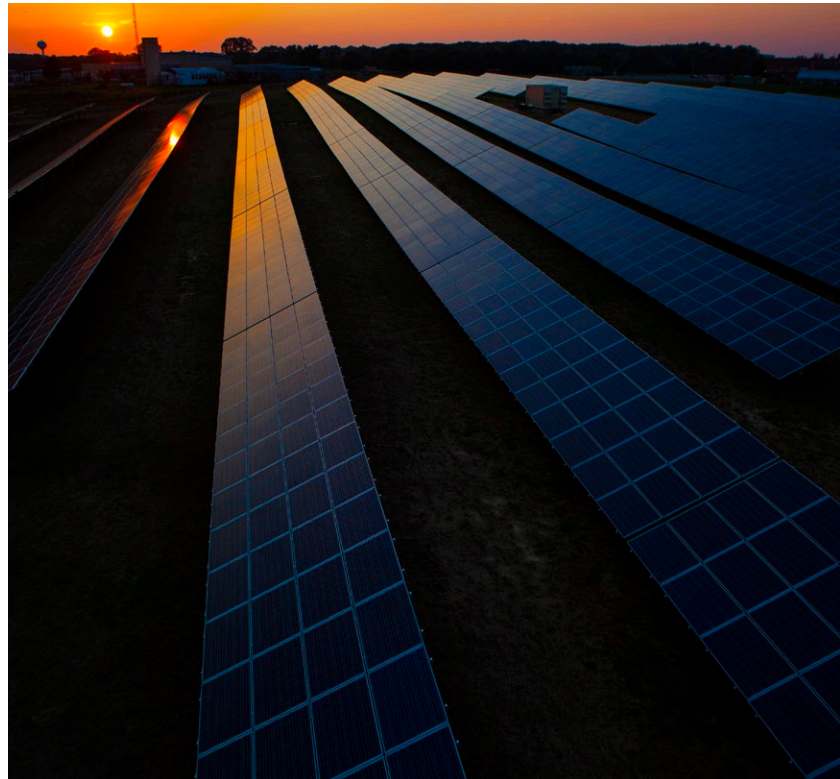
Ground mount installation in Worton, Maryland
