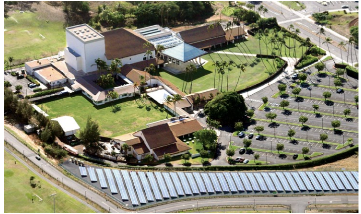
Ground-mount array at Maui Arts Cultural Center in Maui, Hawaii
