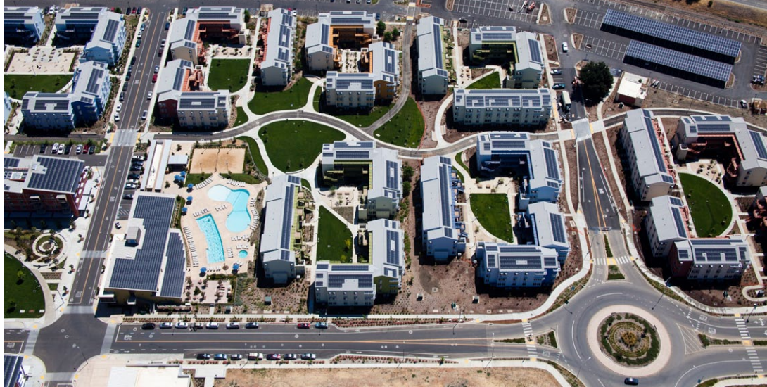
University of California at Davis West Village combines advanced energy efficient design features with a 4MW high efficiency SunPower solar system. It is the largest zero net energy development in the nation.
