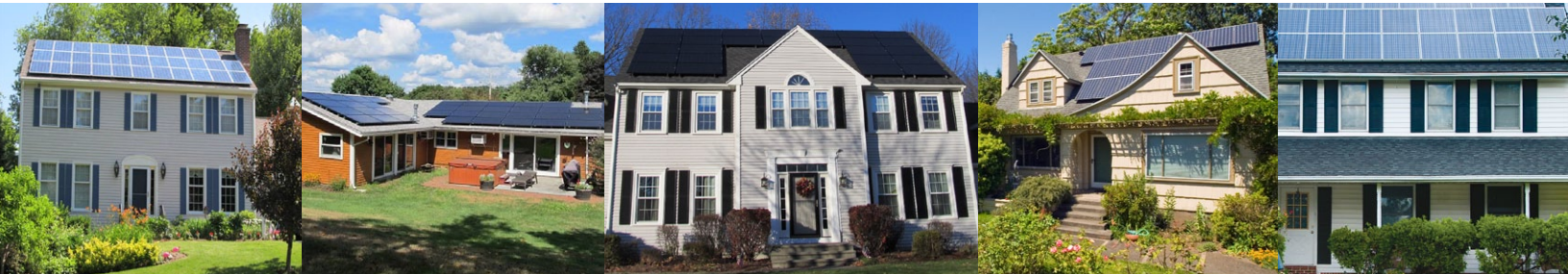
Residential PV Installations
