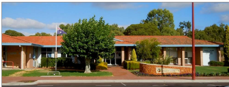
Shire of Capel Administration Centre
