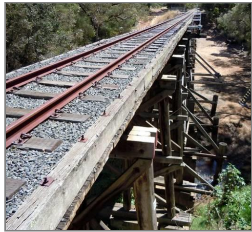
Timber rail bridge over Capel River
