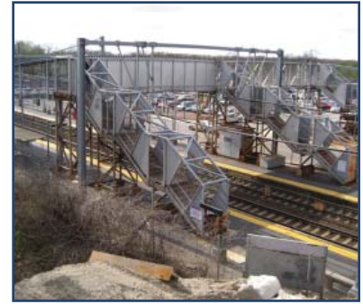
Figure 10-5: Several Views of South Attleboro Station
