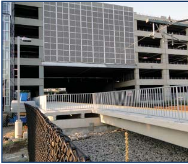
Figure 10-3: T.F. Green Airport commuter rail station and connecting skyway
