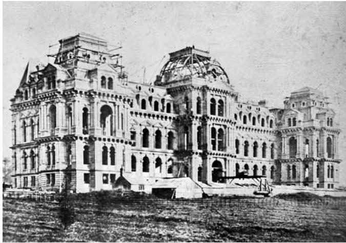
100 This remarkable photograph, taken in early 1876, shows the main structure of The Bowes Museum nearing completion, with only the windows and great dome still open to the skies. Just visible on the central dome is a minute figure.
