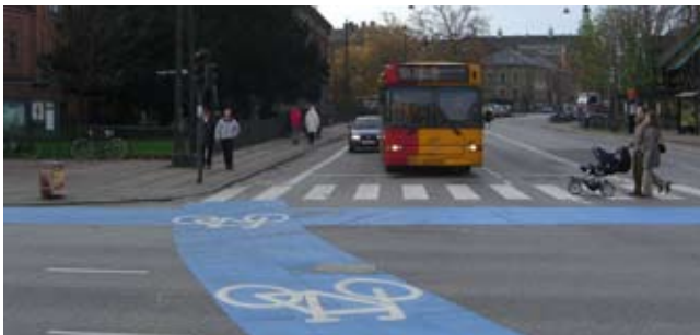
Tietgensgade and H.C. Andersens Boulevard is an example of a truncated track with a narrow painted lane to the intersection with an advanced stop and blue crossing.
