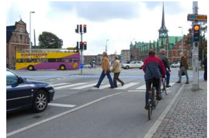
The intersection of Vindebrogade at Holmens Bro is an example of a track to the intersection with an advanced stop but no marked crossing. The stop line for cars has been withdrawn five meters from the pedestrian crossing, which adds to the intersection safety both by making drivers more aware of bicyclists and by giving bicyclists a head start across the intersection.
