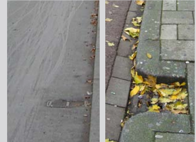
Copenhagen's grate design causes cyclists to weave to avoid grates, especially when they have sunk into the ground (above, left). An Amsterdam cycle route highlights an effective alternative grate design (above, right).
