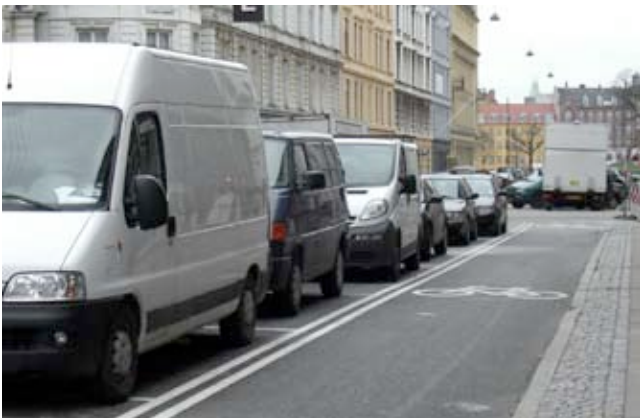
At Vendersgade, a contra-flow lane has been installed along the one-way street, which has two white lines and bicycle symbols to distinguish it as a bicycle path.
