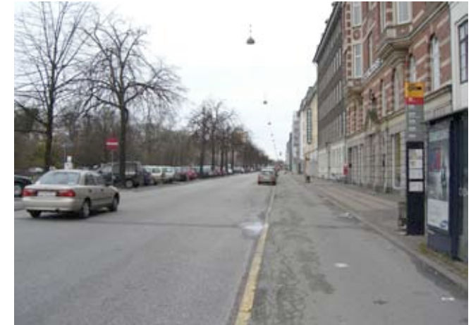
Along Nørre Voldgade, a bus stop is adjacent to the cycle track. Where cycle tracks are provided, most accidents occur between bus patrons and cyclists. When the bus delivers passengers directly onto the cycle track, cyclists must yield the right-of-way, which can slow down travel time. Painting zebra crossings on the cycle track can be effective at reducing the traveling speed of cyclists.
