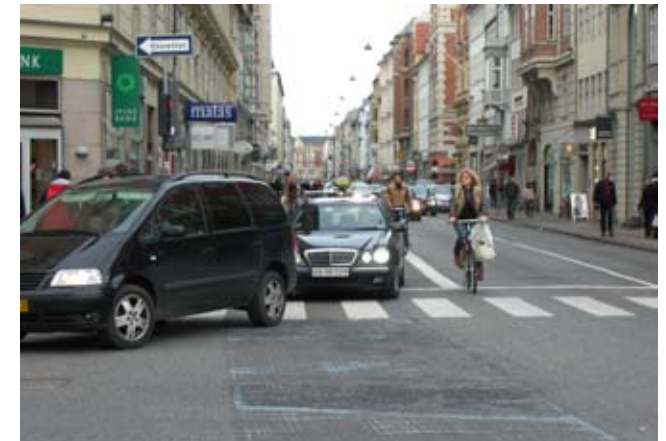
At Gothersgade and Store Kongensgade, a bus priority project has changed the design from an advanced cycle stop and a lane up to the intersection to a shared design. Remnants of a blue-marked crossing are visible.
