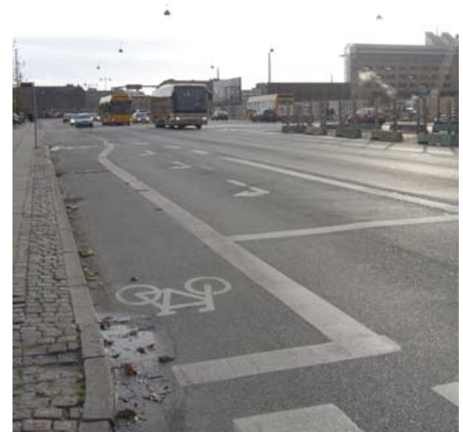
The new standard design for intersections in Copenhagen, will incorporate a painted cycle lane up to the junction.
