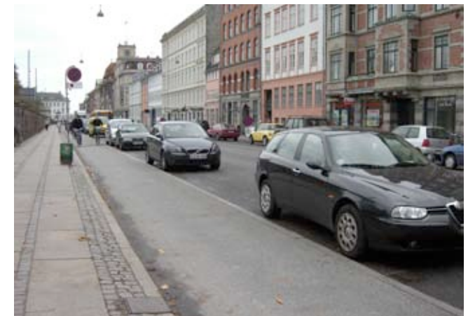
The typical Copenhagen cycle track with adjacent parking, here along Gothersgade.
