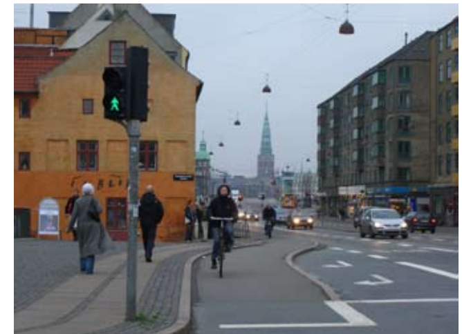
Along Torvegade near the Christianshavn Metro, an advance stop reduces conflicts with right-turning cars.
