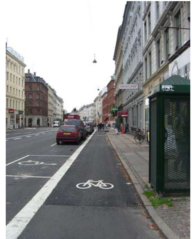
Nørre Farimagsgade near Frederiksborggade incorporates parking with painted spaces so cars know where they belong. The painted lanes are typically the same width as a cycle track, at 2.2 meters. The white stripe is 0.3 meters wide and continuous, except for junctions with side roads, where it is broken to indicate the presence of cars. Bicycle symbols should be placed every 100 m and after junctions (Jensen, 2000).
