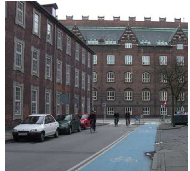
A contra-flow lane on the Strædet route near Vester Voldgade provides space for cyclists traveling against cars.
