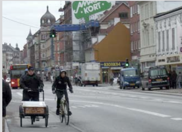
Along Amagerbroagde, a bicyclist must ride very close to the edge of the cycle track in order to pass a cyclist on a three-wheeled bicycle. This can feel quite uncomfortable, but so does traveling at a slower than desired speed.
