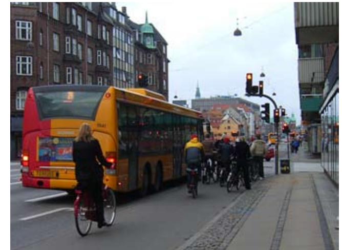
At Torvegade and Prinsessegade, the junction features bicycle light that has separate straight and right-turn functions. Since the track does not feature separate lanes for cyclists, right-turning cyclists either wait for straight-on cyclists to go, weave into traffic, or bike on the sidewalk.
