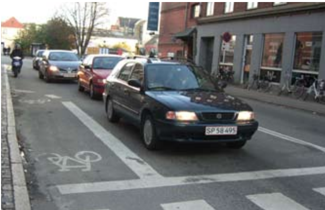
When Øresundvej, a mixed street, meets the major junction with Amagerbrogade, it has a short cycle lane.
