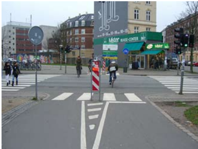
Where the Nørrebro route meets major roads, the junction is usually signaled, like this one above at Nørrebrogade. Road signs, painting, and rumble strips give cyclists a heads up about the approaching intersection as well.
