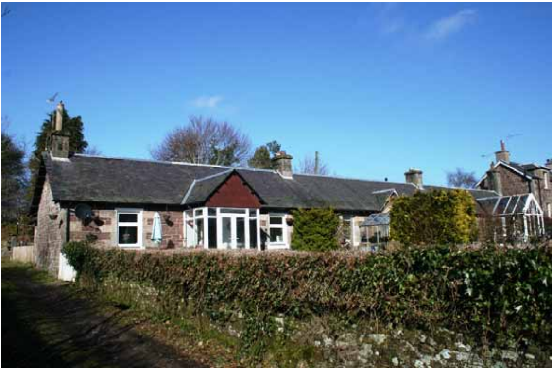
Fig 8: adjoining The Steading, The Cottages continue the more rural, less formal feel of the southern end of the village. A low row of 3 houses with long front gardens enclosed by hedging and stone boundary walls. Two of the original small gabled entrances have been extended with entrance porches which are not part of the original design.
