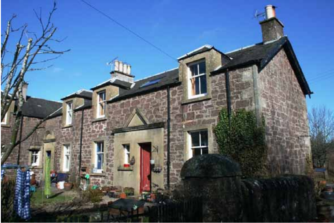
Fig 7: west elevation of The Steading; the houses in the southern section of the village were designed for different uses and this is reflected in their architectural style although there is a continuity in the use of materials such as the red sandstone. Note the eaves dormers and distinctive door surrounds with small pediments over.
