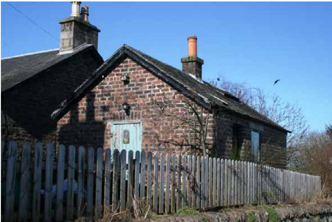
Fig 6: outbuildings, originally wash houses, privies or coal sheds, form an important contribution to the character of the conservation area and are an integral part of the planned model village. They are constructed in brick, but maintain the architectural detail of the cottages such as segmental arches over openings.
