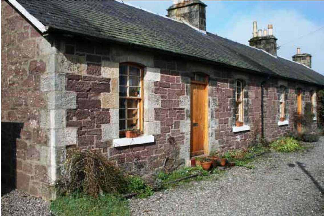
Fig 5: detail of one of the cottages of The Square with a carved stone 'Gladstone Square 1868'. This unaltered cottage illustrates all the characteristics of the original houses: contrasting red and cream sandstone, segmental window and door lintels, 6 over 6 laying pane timber sash and case windows (originally painted finish), boarded door with 2 pane lay-light and small planting strip in front of the cottage. The quality of materials and attention to detail illustrate Pullars intention to construct an attractive factory village.
