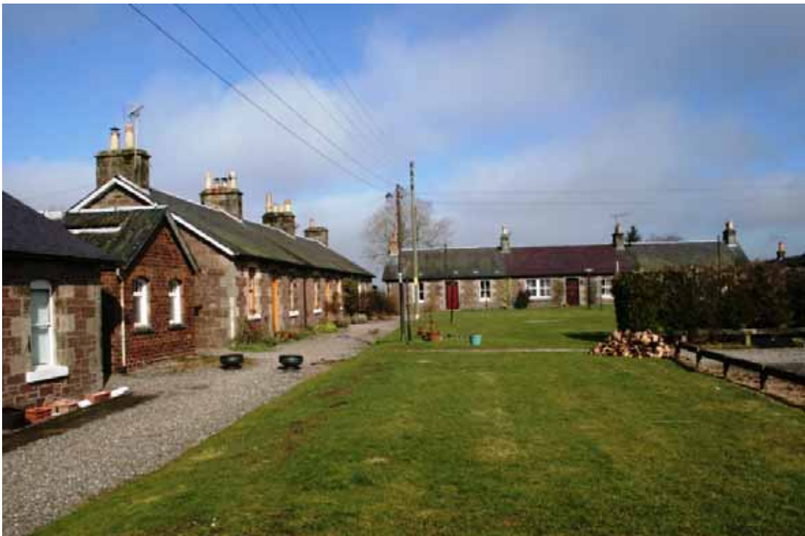
Fig 2: view looking north-east across The Square. The single storey cottages in groups of three 3-bay houses form a U plan around a communal drying green. Note the small brick building on the right, one of several former wash houses, privies and coal sheds which remain an integral part of the planned village.
