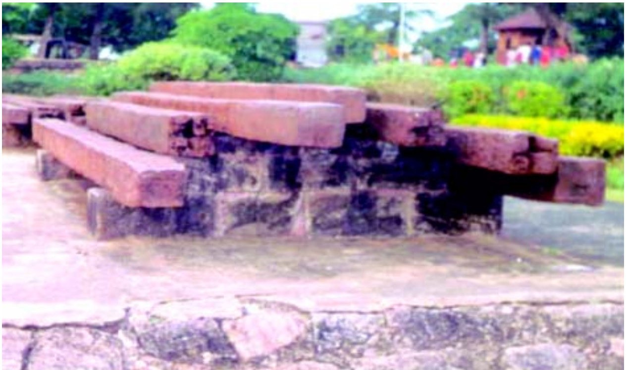
Fig.16: Iron beams in Konarak Sun temple placed on supports in the courtyard.
