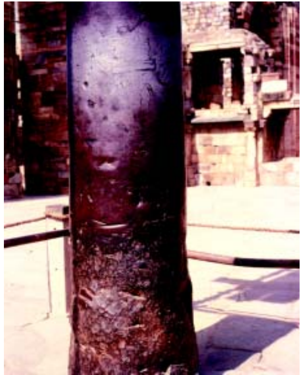
Fig.6: Bottom region of the iron pillar. The rough portion was originally buried in the ground.
