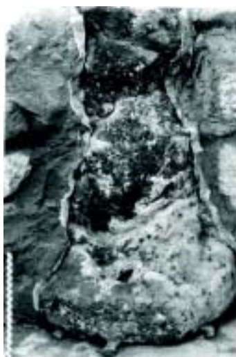
Fig.8: The underground portion of the pillar below the ground level after provision of a new lead coating before being buried again in 1961.
