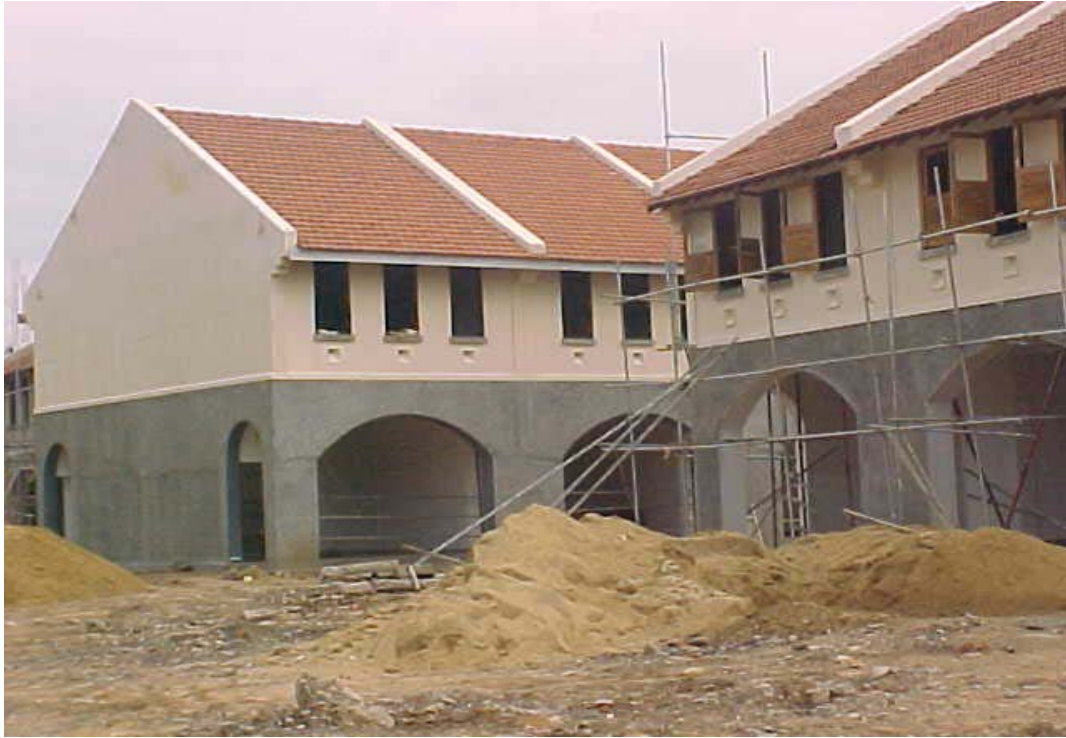
Construction of Shop houses at Pettigalawatta
