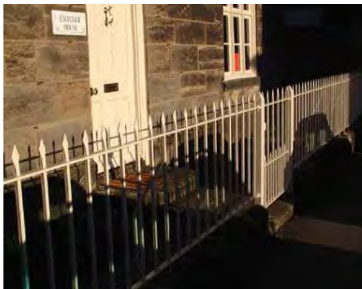
Below right - hand-forged railings in steel; a modern interpretation of wrought ironwork by David Tucker (11 Blanch Croft)
