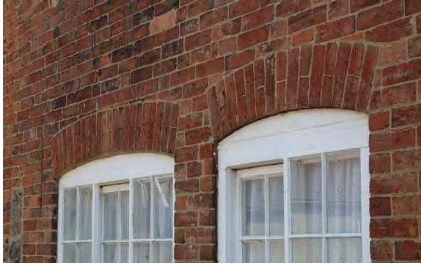
Left - where economy was important, lintels were simpler in form; a segmental arch formed by "stretcher and header" bricks (18 Market Place).
