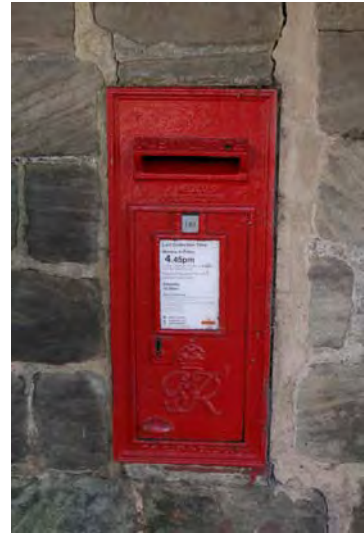
Right - Wall-mounted letter box (GR). Blackwell Lane, on north wall of Melbourne Hall estate yard
