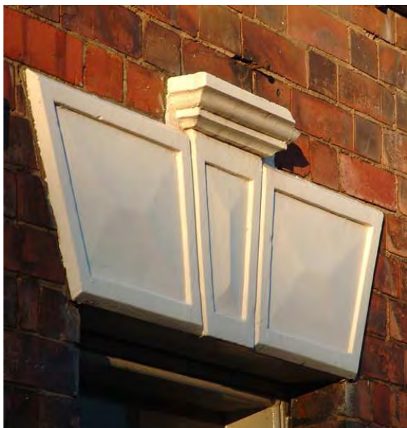
Left - stone wedge lintel at High Street designed to look like panelled timber with raised and fielded panels. Above - (top to bottom) 15 Potter Street; 7 Potter Street; Close House; 55 Penn Lane.
