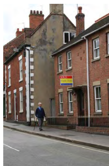
Alterations to building line
