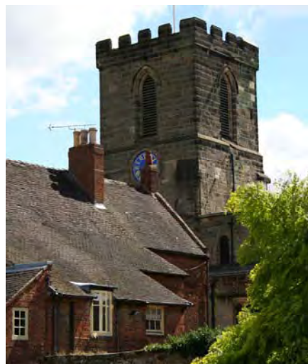
Church from Church Street
