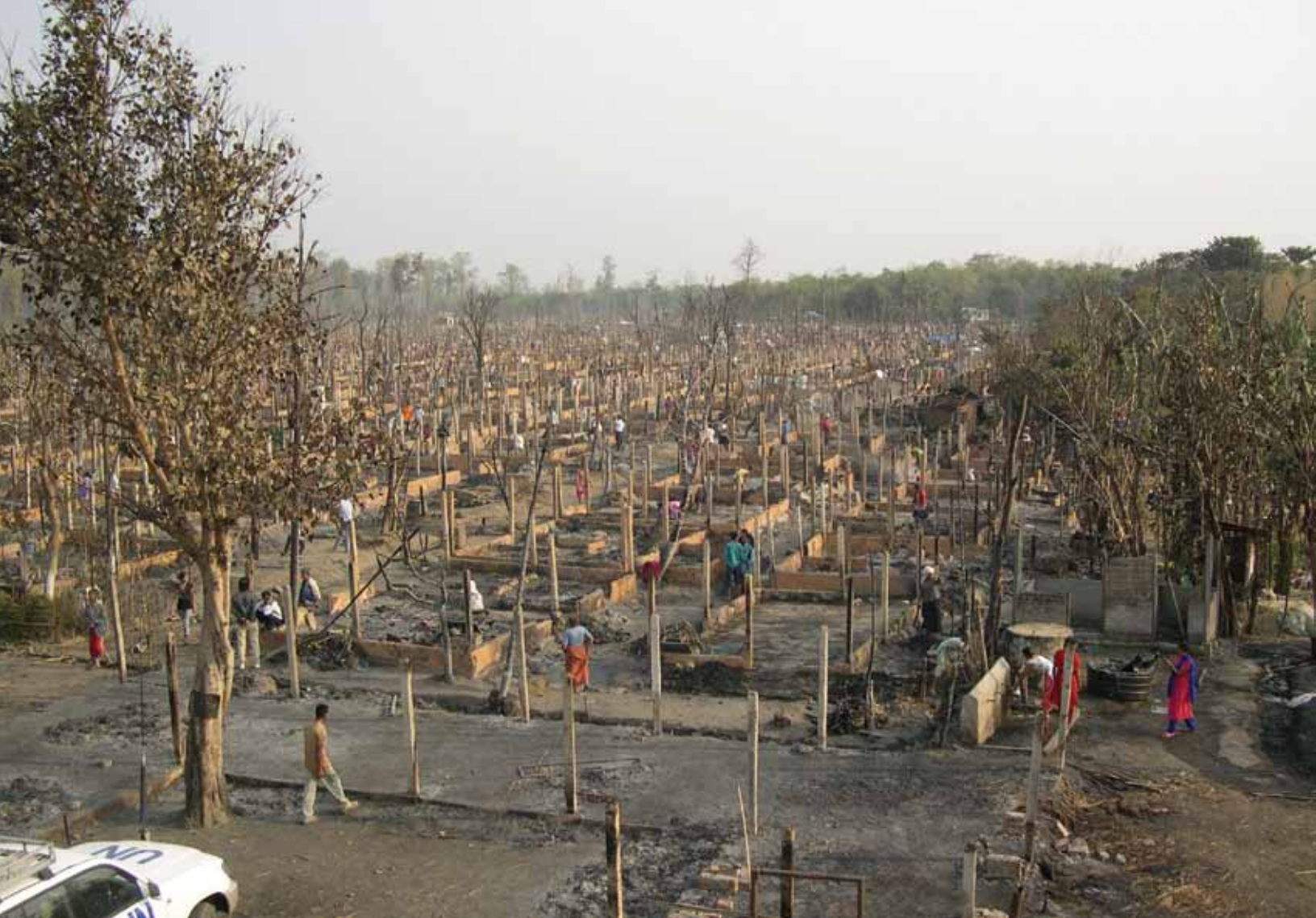
Nepal's Goldhap refugee camp in the wake of a March 2008 fire. Nepal does not allow electricity in the camps, forcing refugees to use open flames for cooking, heating, and lighting. Credit: UNHCR
