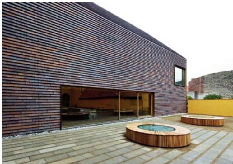
Sorø Museum is covered by a dark-red, clinker-built Kolumba K43.
