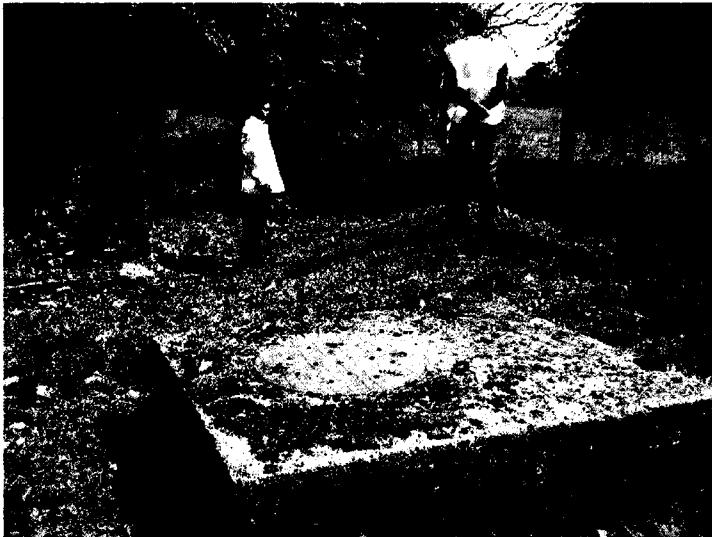
Figure 1. Photograph of manhole that overflows (ref. SW3) due to hydraulic limitations of sewer.
