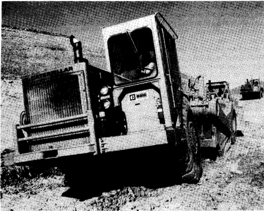
Scrapers at work at McDermitt Mine.
