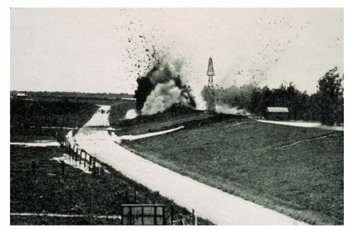
Figure 4: Dynamiting of the levee at Caernarvon, Louisiana to take pressure off levees further upstream at New Orleans (Courtesy of NOAA's National Weather Service Collection)
