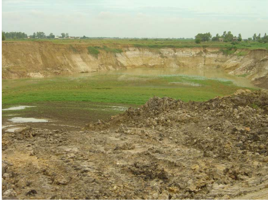
Photo 5: Excavation of Boeung Pong Peay
