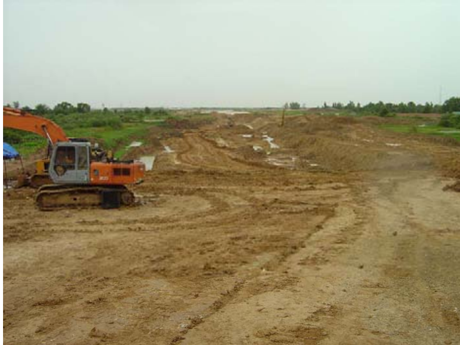
Photo 3: Construction of the Grand Canal du Nord
