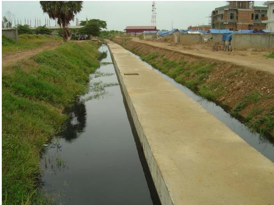
Photo 6: Construction of Tuol Kork Canal to Oveng Canal Drainage Link
