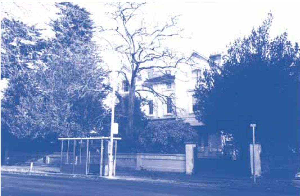
Photo Six and Seven: Mansfield Hall
