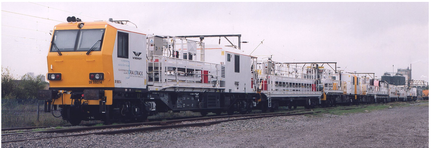
High Output Wiring Train – Full Consist
