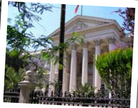
The Former National Congress Building, Santiago
