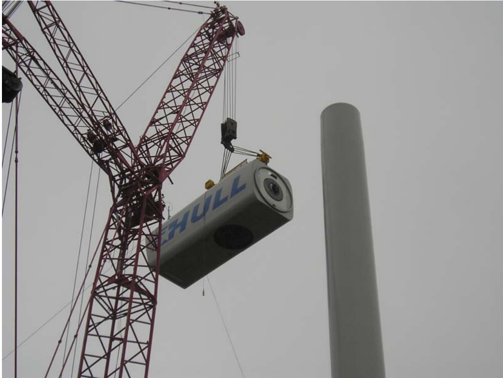
Figure 15 Nacelle Installation
