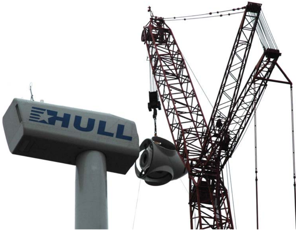
Figure 16 Hub Installation
