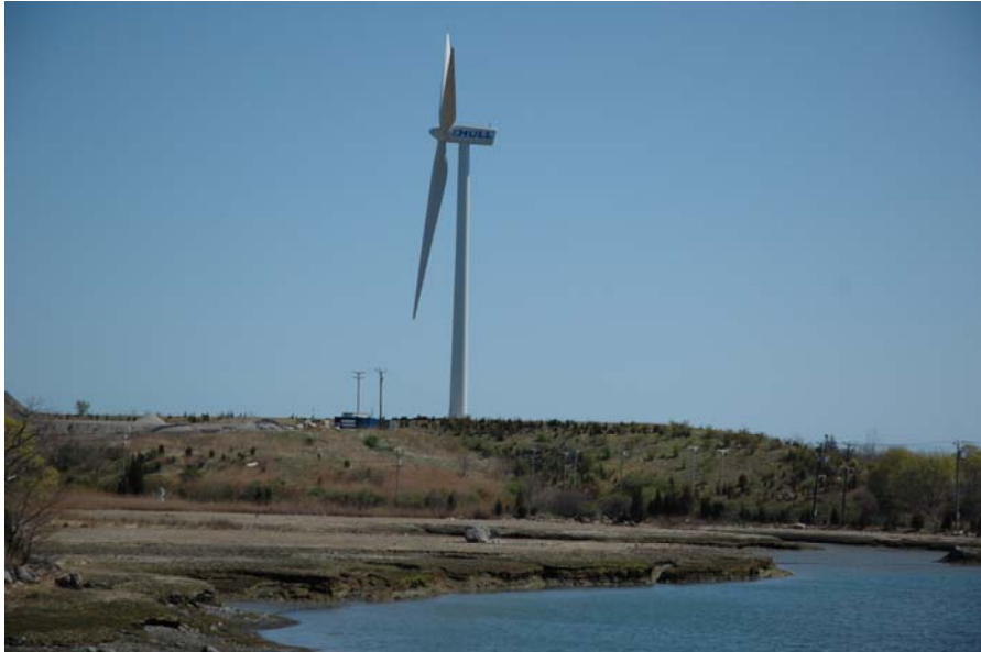
Figure 19 Hull Wind II Installation Completed
