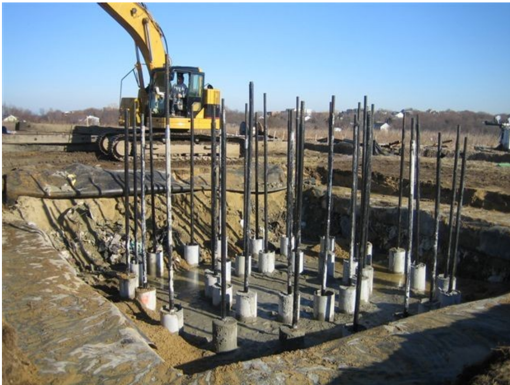
Figure 12 Piles and Rock Anchor Bolts for Hull Wind II Foundation
