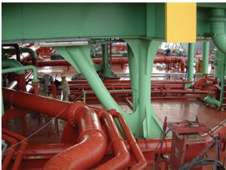
Figure 3-3: Topside support welded directly to deck
