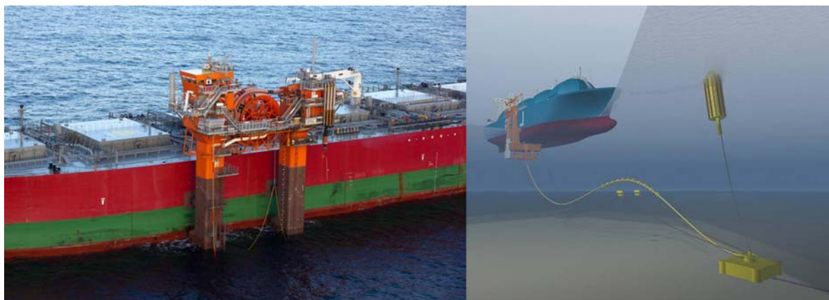
Figure 4-24: Torp LNG Transfer system – Courtesy Remora
