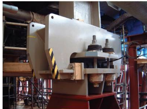
Figure 3-5: Topside support on sliding support
