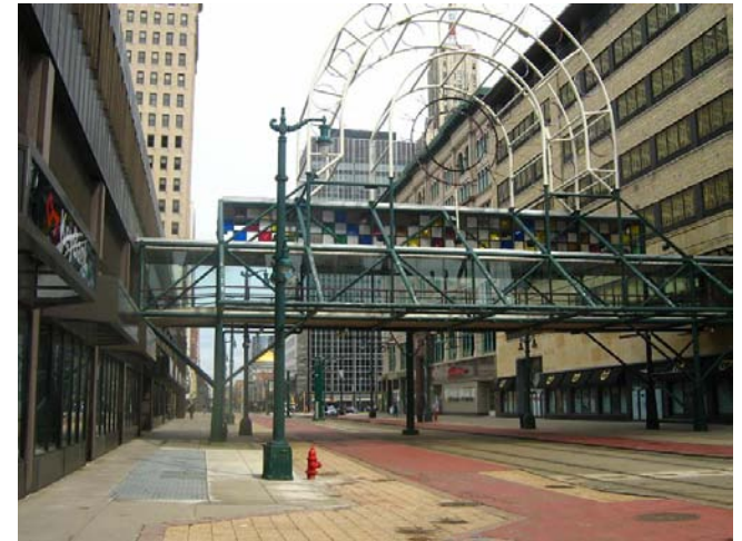
FIGURE 4: Buffalo, New York's failed Main Street Mall (Source: metrobuffalo.com)
