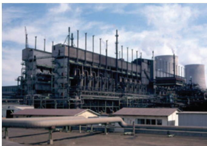
FIGURE 2 Lurgi Gasifiers in Secunda, South Africa
