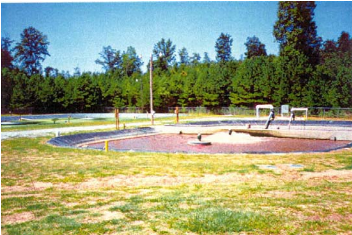
Reactor basin with first cell in foreground
