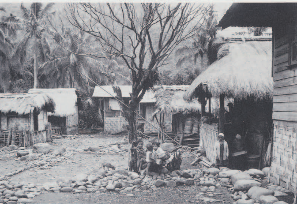
Figure 3b. Typical scene within the village of Dangtalan. Traditionally, Kalinga houses are built several feet above the ground. Construction materials include split bamboo and cogon grass. Galvanized iron roofing has recently become a popular alternative to thatched roofs. Costly to obtain, metal roofing is more resistant to damage during monsoon storms, but it also conducts heat from the tropical sun and makes for warm house interiors.
