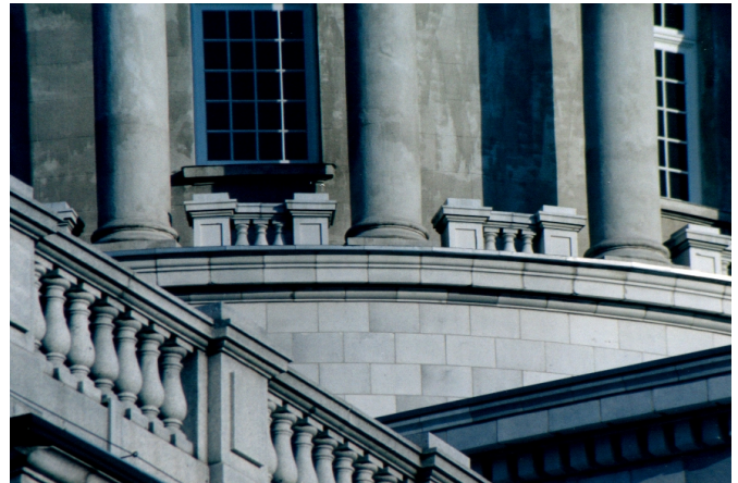
ROOF INTERSECTION OF PARAPET BALUSTRADE.
