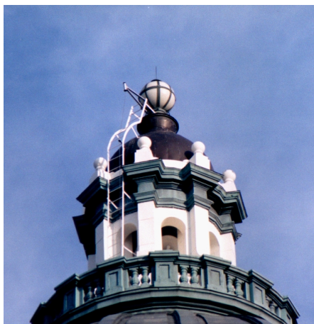
WHITE PAINTED METAL ON LANTERN, ABOVE DOME
