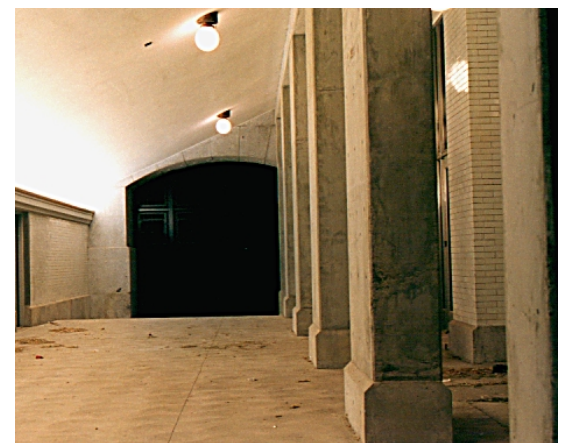
GROUND LEVEL SOUTH ENTRANCE UNDER GRAND STAIR
