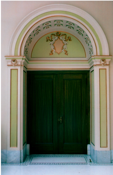
DOOR DETAIL, FOURTH FLOOR CORRIDOR
