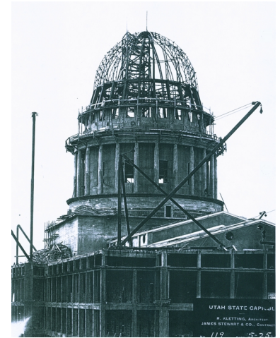
DOMES UNDER CONSTRUCTION
