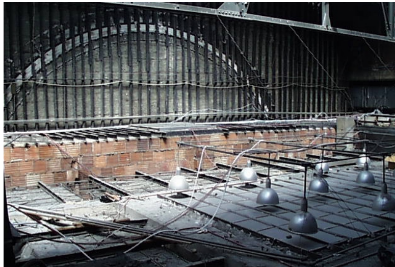
SUPREME COURT ATTIC SPACE, ABOVE THE SKYLIGHT
