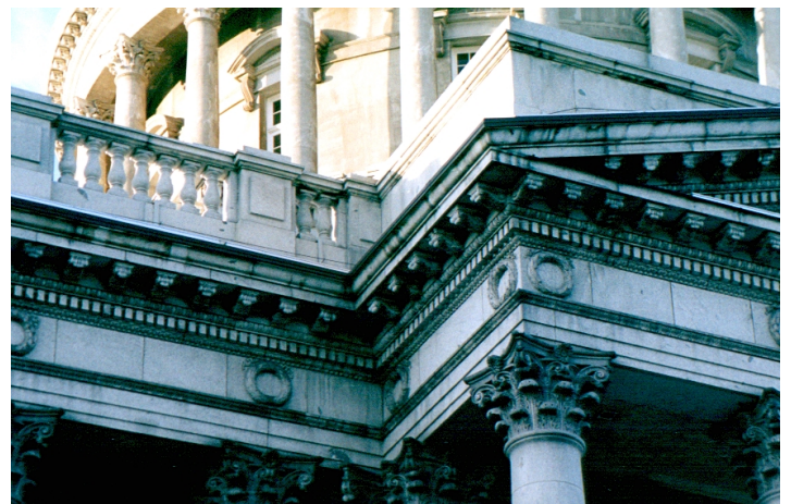
PARAPET BALUSTRADE MEETING ENTRY PORCH PEDIMENT
