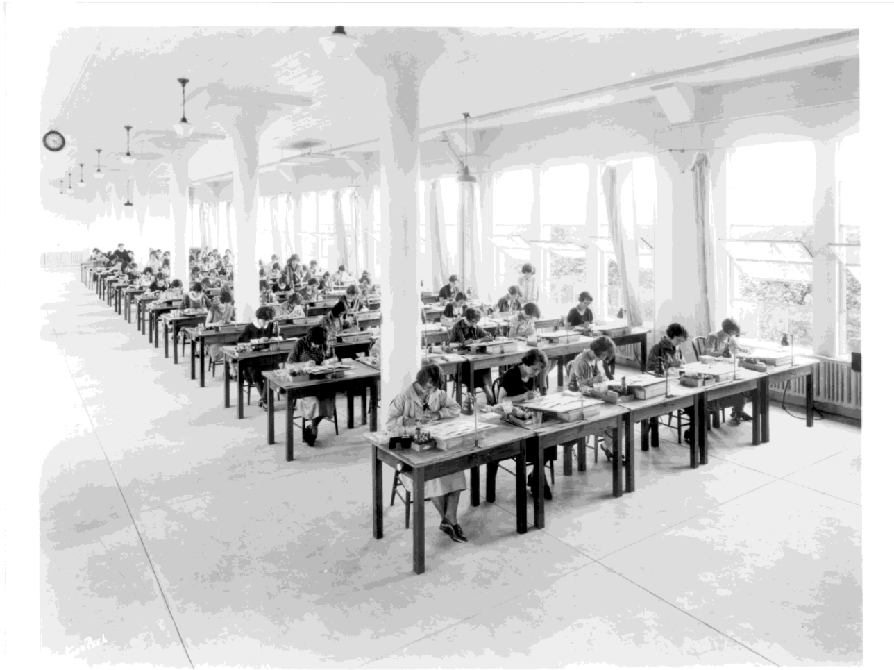
Figure 7: Historic image, Buzza Company Building, interior of factory floor, ca. 1927. (Hennepin County Library, Minneapolis)
