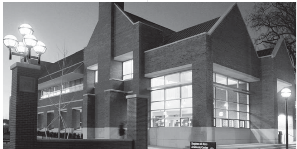
The Stephen M. Ross Academic Center is the academic home for varsity athletes at the University of Michigan. Completed in winter 2006, this $12 million, 38,000-square foot building provides academic study space for more than 700 U-M student-athletes. The three-floor facility is situated adjacent to Yost Ice Arena.
