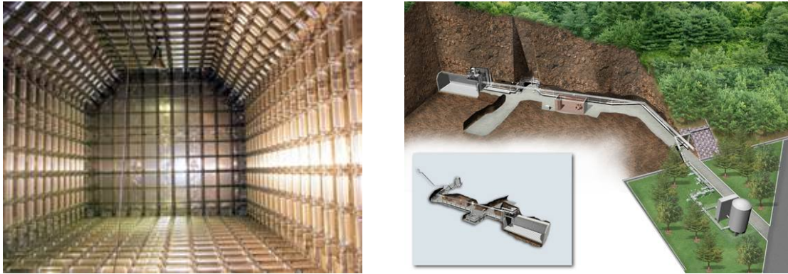
Figure 9. Application of the membrane technology to cryogenic caverns
