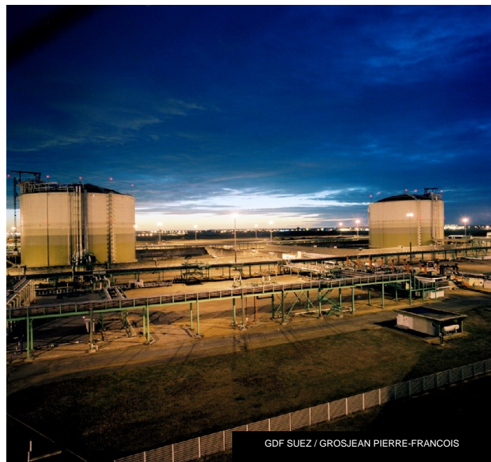
Figure 1. The two first membrane tanks at Montoir-de-Bretagne
