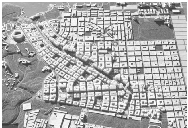
Credit : Julio César Pérez Hernández et al. (Source : p. 71 of Master Plan Doc)
