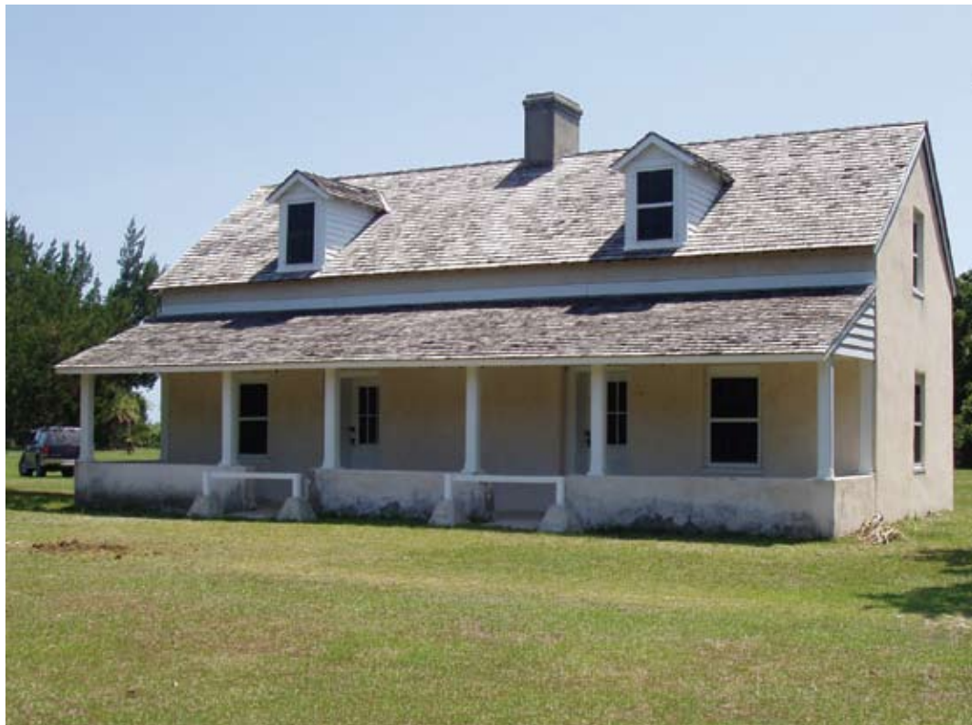
Located within the Dungeness Historic District, the Tabby House originally served as a caretaker's residence. The house was named after its construction material. Tabby was an early predecessor to cement, made by mixing lime, sand, and sea shells.
