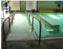
Figure 20. This photograph shows the entrance ramp to a human therapy pool located in a rehabilitation hospital in a metropolitan area. This ramp or beach-type entrance allows easier access for many patients. The water is typically maintained around 92 degrees F. It remains to be seen if therapists in the future will be allowed access to such pools for canine patients. Some of the major issues are concerns regarding control of infectious agents and maintenance of water quality. (Courtesy of Cheryl Fuller, MS, ATC, Aquatics Director, Spain Rehabilitation Center, The University of Alabama at Birmingham). - To view
