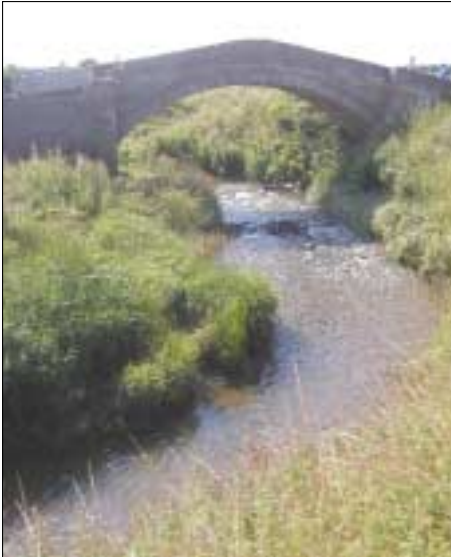
Bridge over the River Blyth
