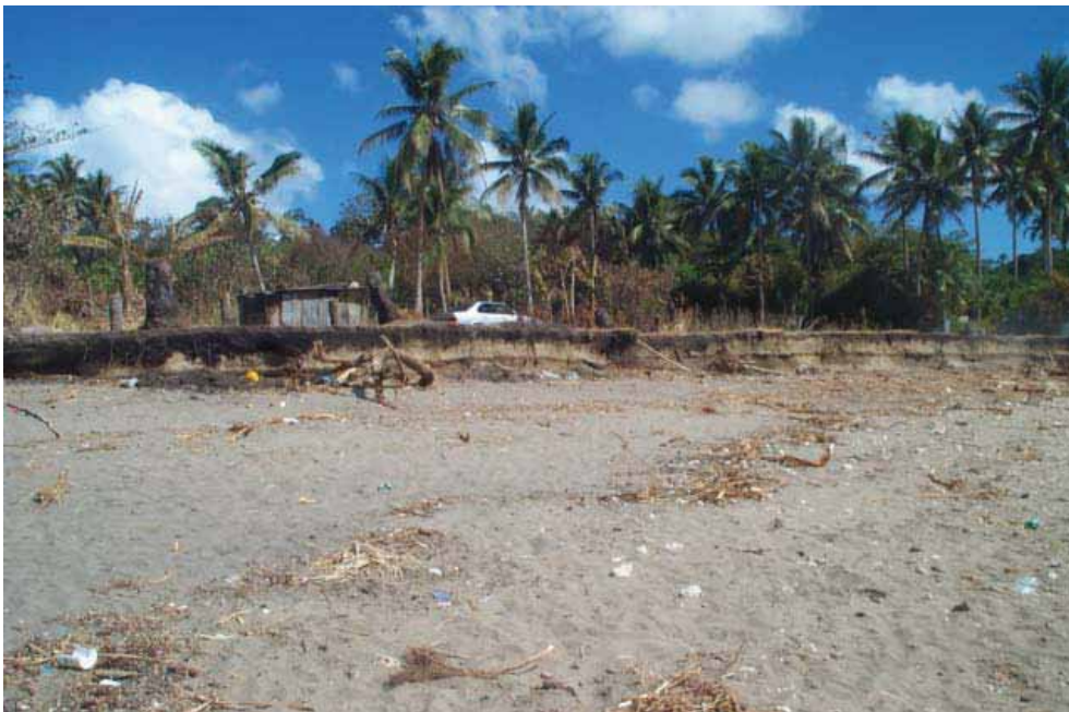
Figure 6: Location 3. Erosion of bank and over-topping
