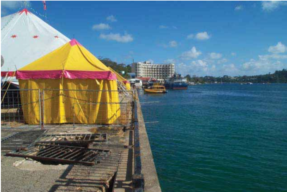
Figure 5: Location 2. Over-topping of the sea wall
