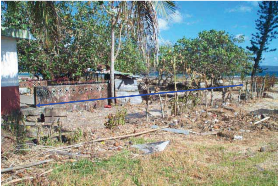
Figure 7: Location 3. Sea water run-up over floor level
