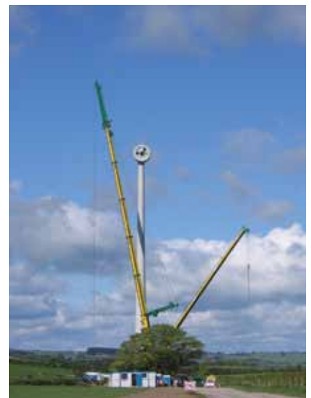
Udney Wind Turbine construction - lifting the hub and blades.
