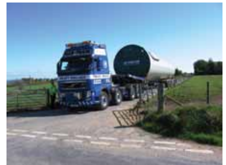
Udney Wind Turbine construction - delivery of tower sections.
