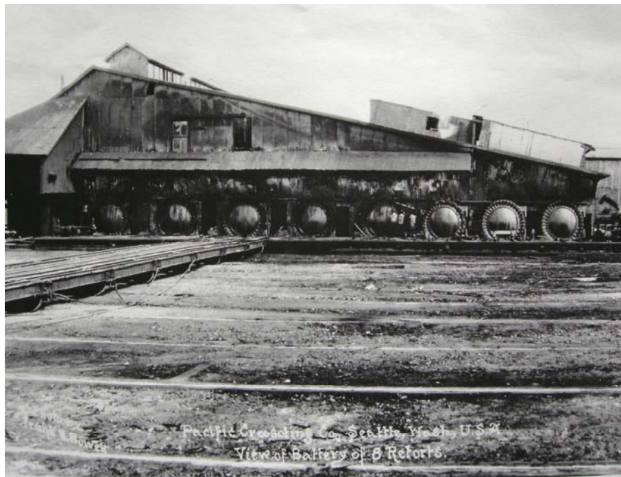
Figure C-3 Retorts to pressurize
