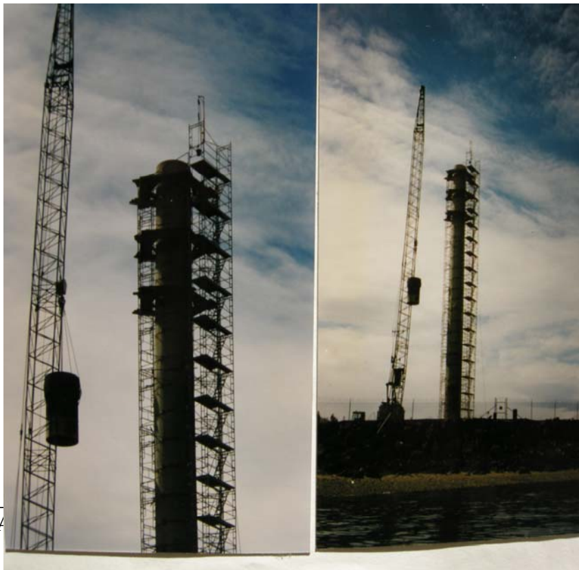
Figure C-8 Removal of the Smokestack
