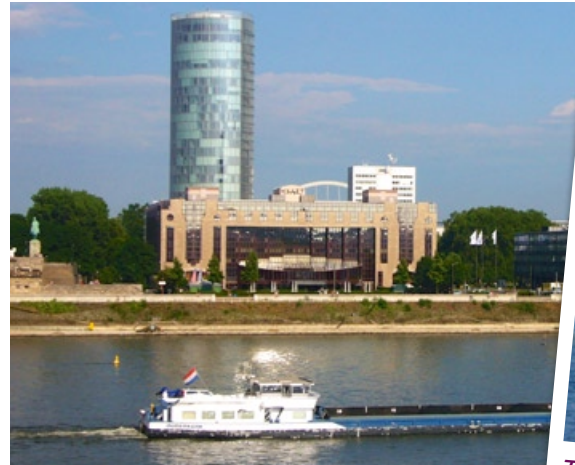
Looking across to the right bank and the 103m Triangle Tower.
