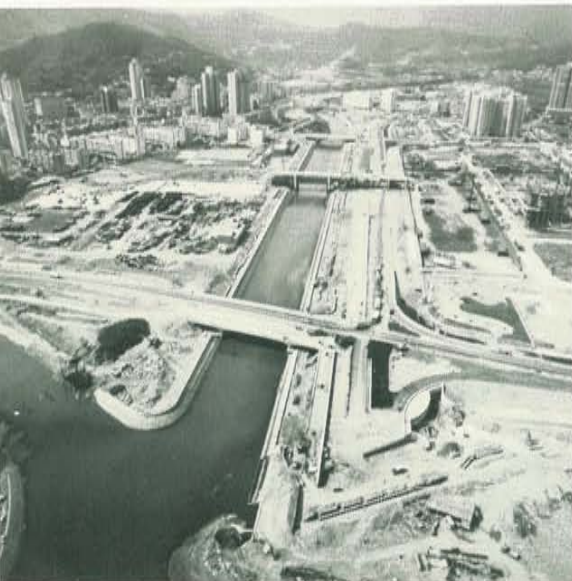
The Tai Po roads and bridges, completed this month.
