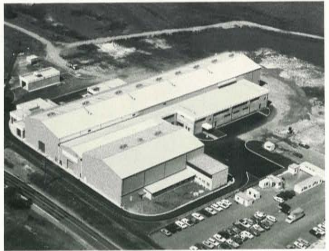
The new boatbuilding factory is located close to Carrington Slipway's main facility, which is one of the largest in Australia.
