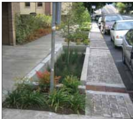
Storm Water Management
