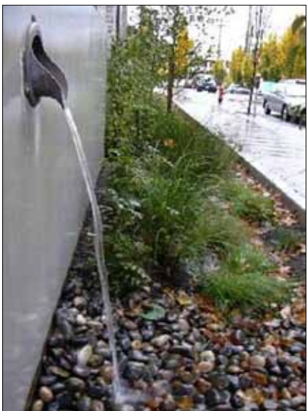
Rooftop Stormwater Treatment
