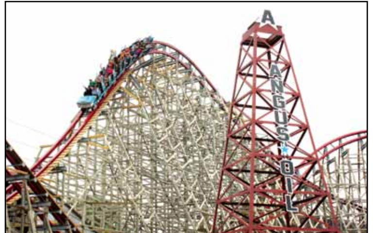
After a 17 month make-over, the New Texas Giant has returned to Six Flags Over Texas, taller, steeper and faster than ever before. The steel tracked, wooden structured hybrid coaster officially opened on April 22. AT / GARY SLADE
