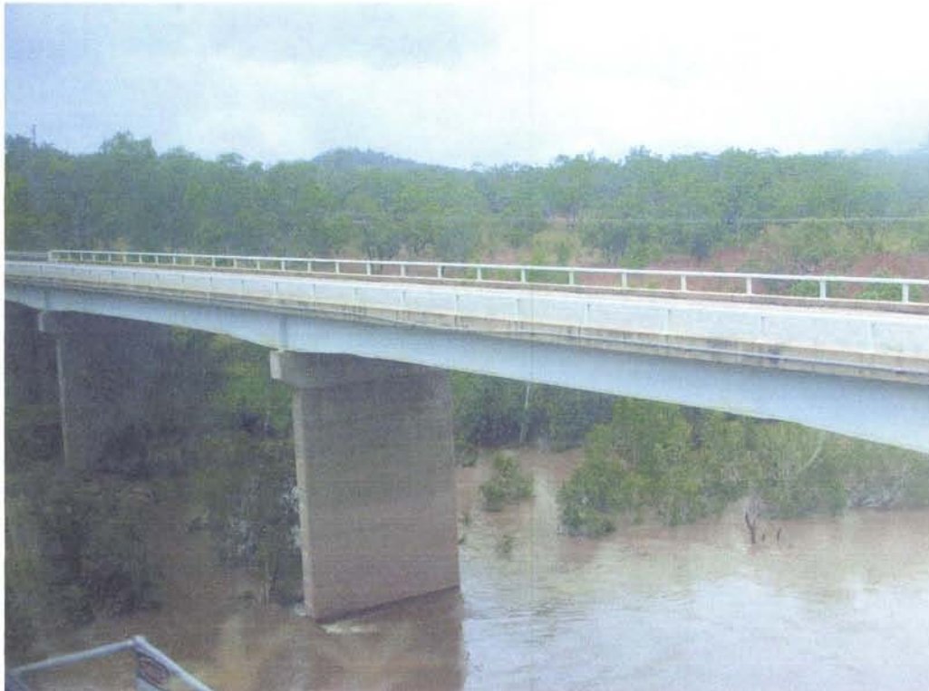
Fergusson River High Level Road Bridge from the Ghan
