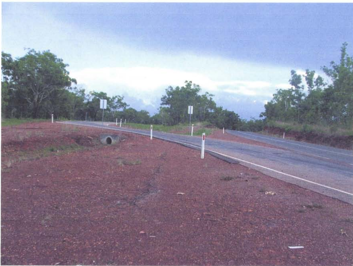
Turn Out to WWII Hwy now used as truck parking bay South of Manton River
