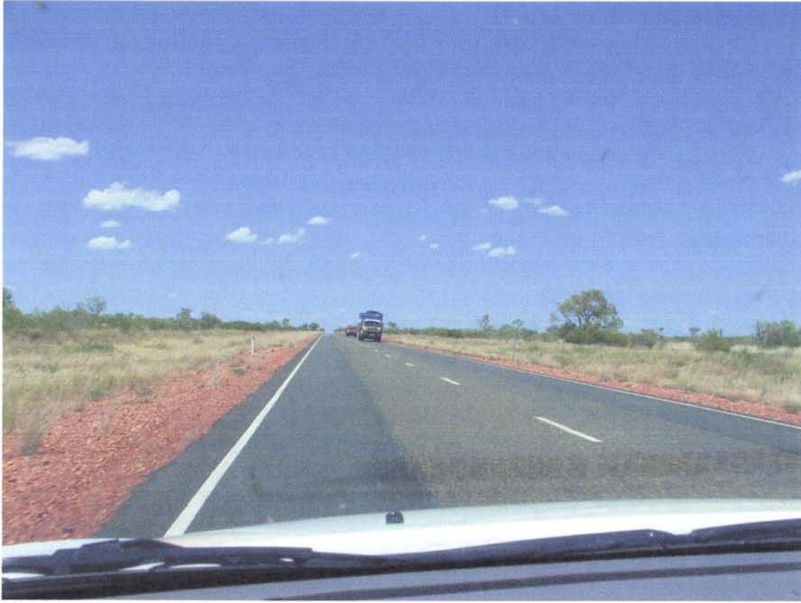
Warrabri Straight WWII pavement upgraded. Widened resheeted
