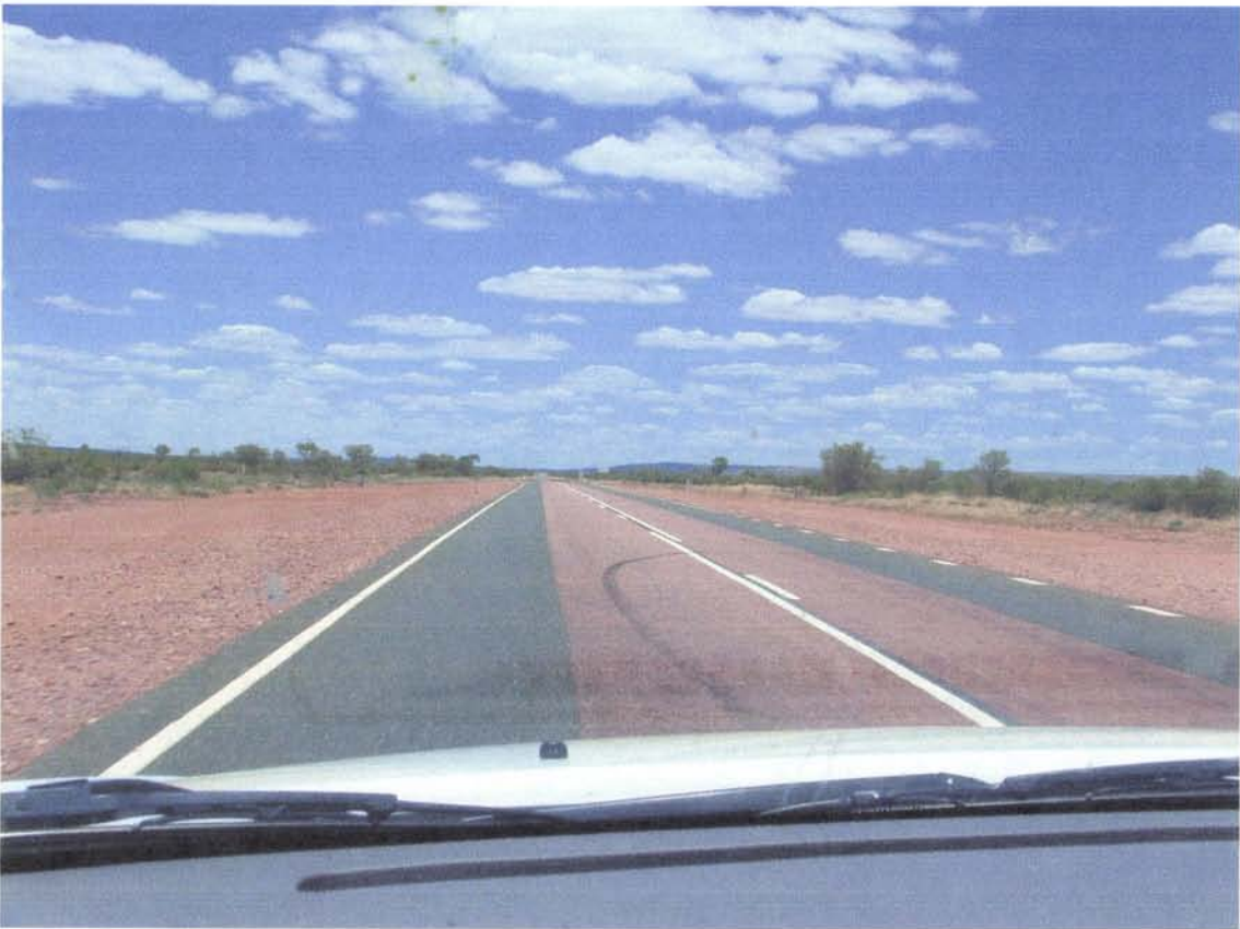
Warrabri Straight WWII pavement widened and resheeted
