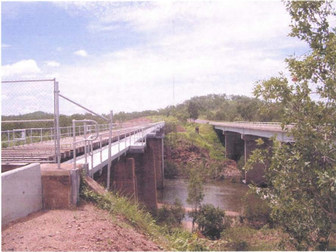
Fergusson River High Level Road & Railway Bridges
