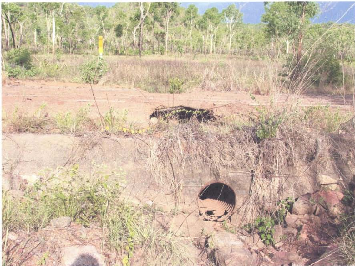
WWII floodway north of Hayes Creek 60 years of weathering Op
