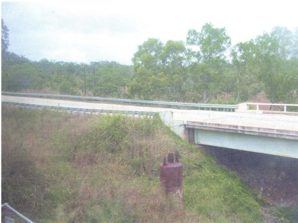
Fergusson River road bridge from the Ghan
