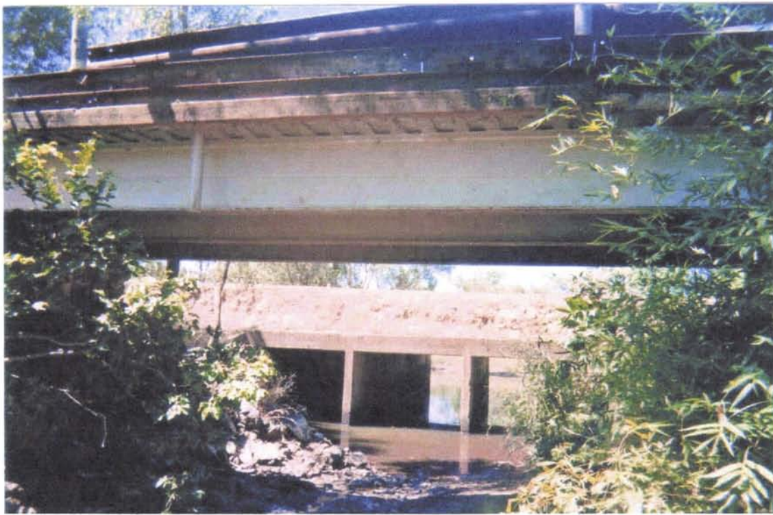
Glenluckie Creek WWII Bridge 1975 Culvert
