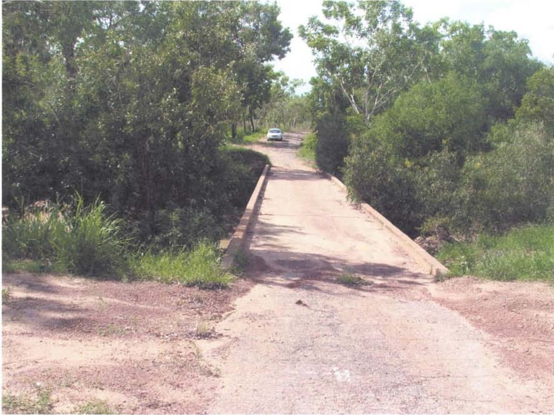
WWII Cullen River Bridge 2
