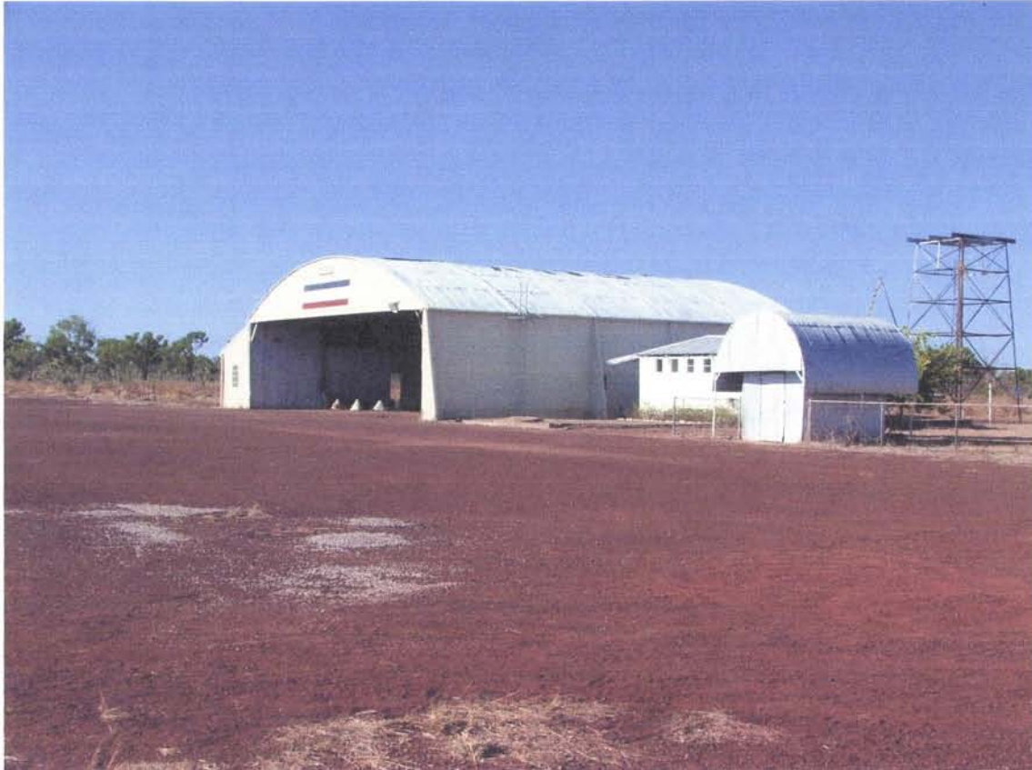
Daly Waters Hangar and Fuel Store
