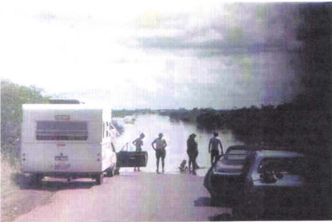
Stuart Hwy WWII Newcastle Waters Creek Causeway April 1975
