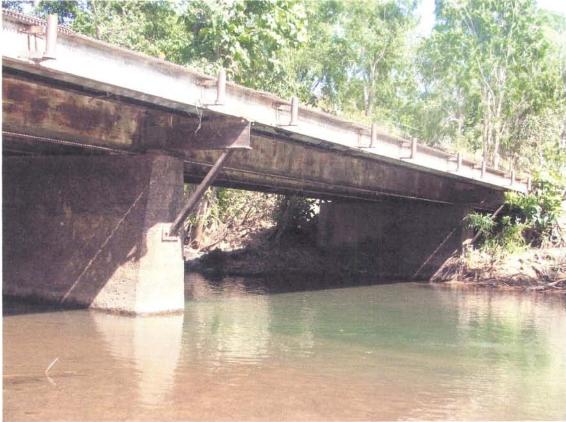
WWII Adelaide River Bridge 1 ARB
