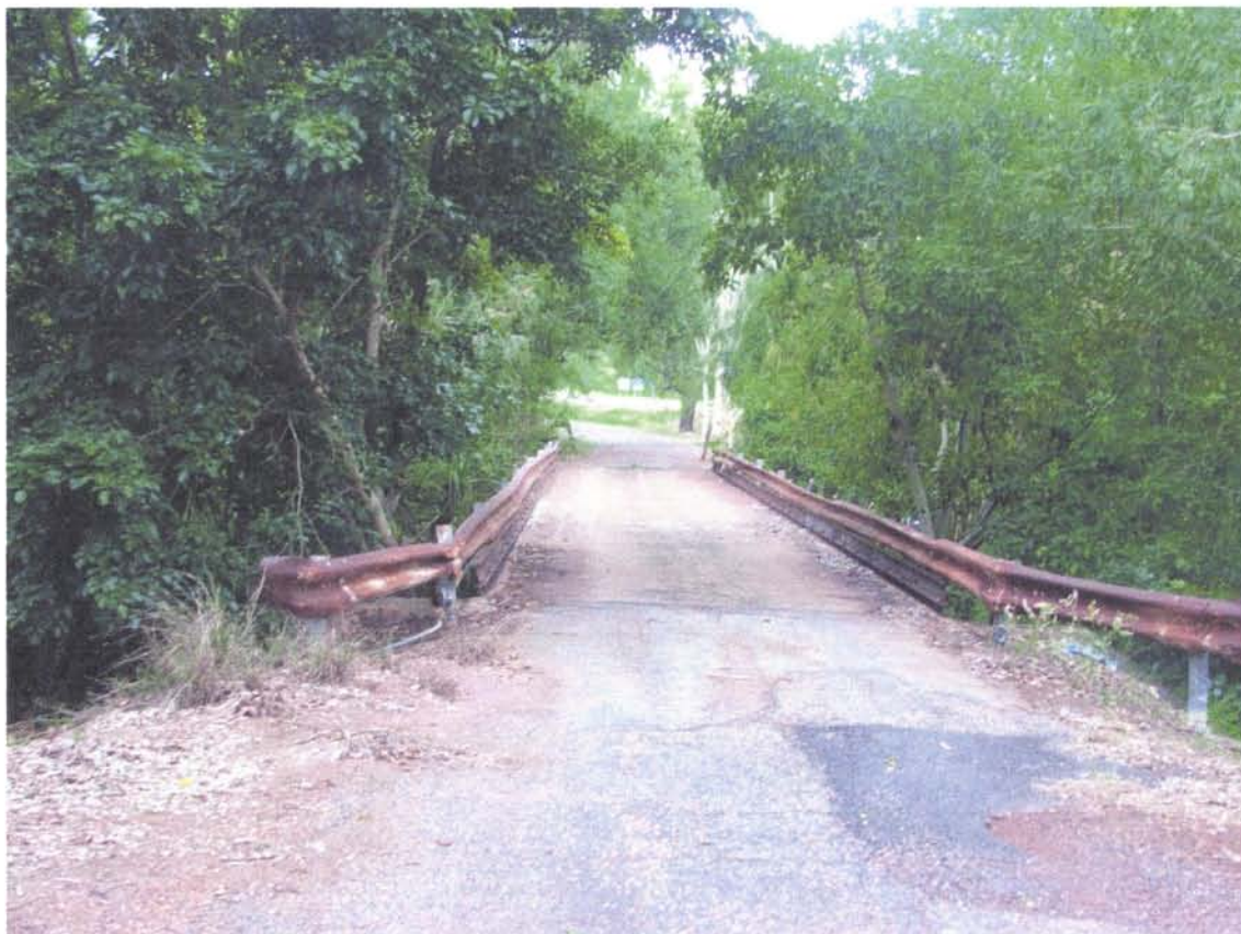
WWII Coomalie Creek Bridge
